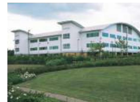
RIGHT - GIVING LAND A NEW LEASE OF LIFE: After acquiring civil engineering company Gilbert Gray we were able to work with the Tyne and Wear Development Corporation. This included remedial work on the former dockyards and colliery sites on the banks of the Tyne (pictured right) and the Wear. As well as work at the Royal Quays, North Shields, St Peter's Basin in Newcastle and Manor Quay, Sunderland - now the site of the University of Sunderland.
